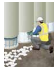
Excavated to basement level, Pilecor is removed and pile reinforcement exposed.
